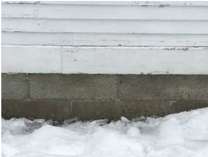
Photo 20: Northwest Foundation: Dressed granite above grade
