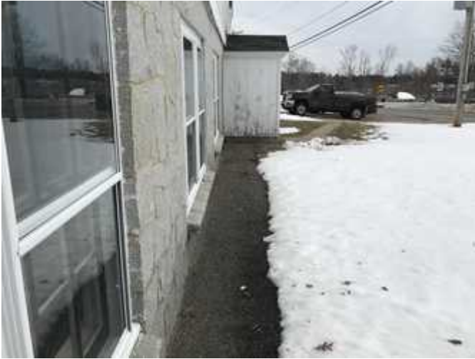
Photo 15: Southeast Foundation: Asphalt drip line
